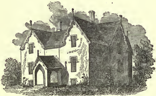
Rectory of St. Peter's Church.
